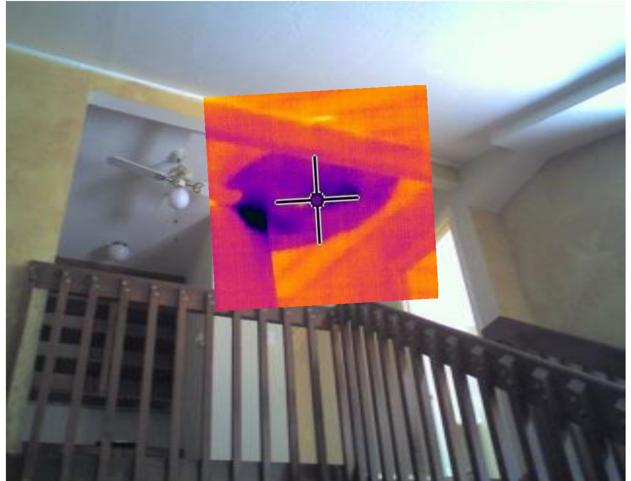
AC condensation leak and clogged drain line caused the drain pan to overflow
