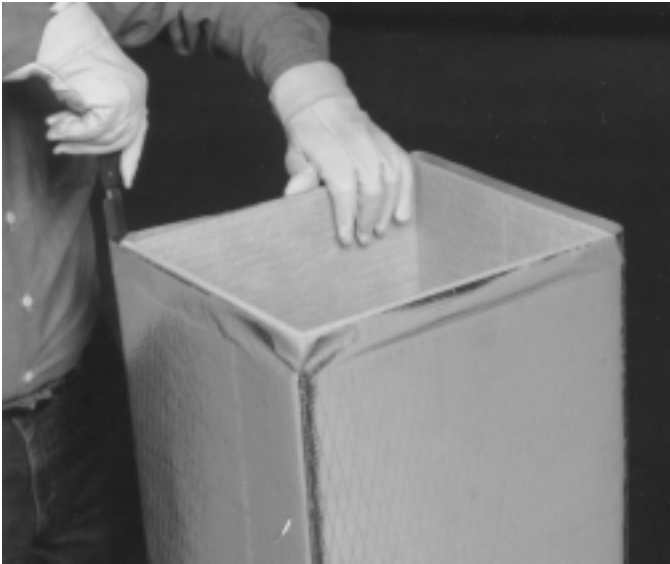
1. Slit facing flaps back at corners, making sure you do not cut below the male shiplap shoulder or into inside duct surfaces.
