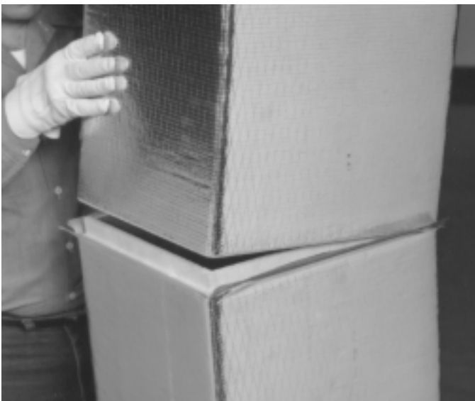
2. Push the two modules together. Make sure male and female shiplaps are tightly fitted together.
