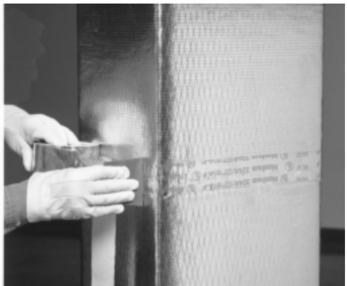
4. Complete closure of circumferential joint with UL 181A listed closure. The minimum width pressure sensitive tape for 1" board is 2 1/2". Three inch tape is recommended for 1 1/2" and required for 2" board. Duct board surface must be clean and dry. (Pressure sensitive tape shown above.)
