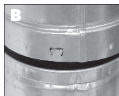
Assemble the gas vent sections
