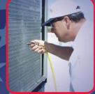
**Blow off coils** with Sludge Sucker® Blowgun
