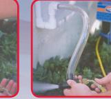
3. Allow Nitrogen to flow through **Sludge Sucker®** fitting and then watch the sludge get sucked out of the drain line and blown onto the ground.
