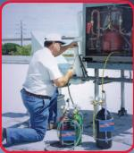
Purge and pressure test an A/C&R system
