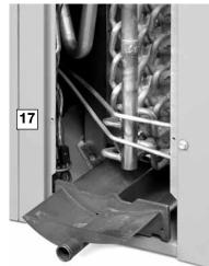
Foil-faced insulation is securely glued and captured to the cabinet. On the base of the unit, closed-cell insulation is used to prevent moisture from being absorbed and help reduce mold content to provide better indoor air quality.
