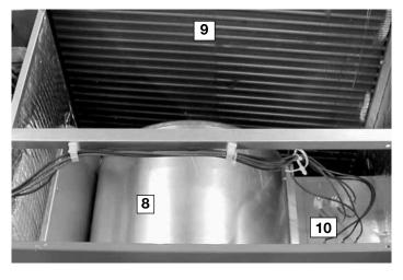
The indoor-section top cover also easily opens to access the removable blower housing and motor (<sup>8</sup>). This also gains total access to the indoor coil for cleaning and service (<sup>9</sup>).
