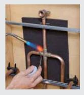
The Insurance Pad is the ultimate heat shield. Use wet or dry, where higher temperature protection and prolonged use is required. Great for use with acetylene air torches. The Insurance Pad delivers protection in excess of 2500°F, an incredible improvement over ceramic and fiberglass heat shields on the market. The Insurance Pad® is a fibrous-felt heat shield with the safest specs in the industry. Repeated use actually increases its heat resistance. Fibers in this heat shield take on graphite
