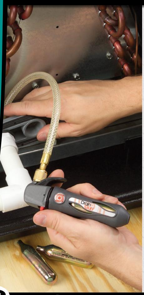
he Drain Gun - Charles Gallo Brand is a lightweight (3oz.) portable tool designed to blow out condensate drain lines instantly. Simply insert a Swoosh CO<sub>2</sub> cartridge into the Charles Gallo Drain Gun and with a press of the trigger — SWOOSH — 800 psi of oil free air clears the line.
